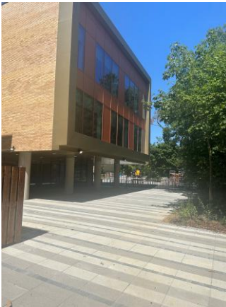
Images show Bletchley post completion, right to left, reclad front façade of existing Andrew Peck building, internal agile teaching space, assembly hub and external of new extension overlooking communal outdoor space
